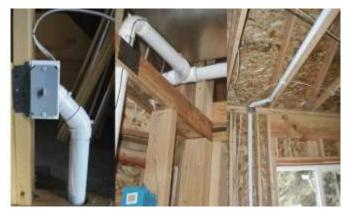
If you can't afford a full system initially, 'plan for the future' by installing the ducting only, at the framing stage of construction.
